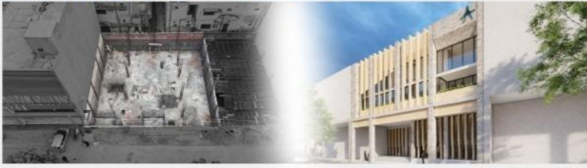
Construction work in progress
